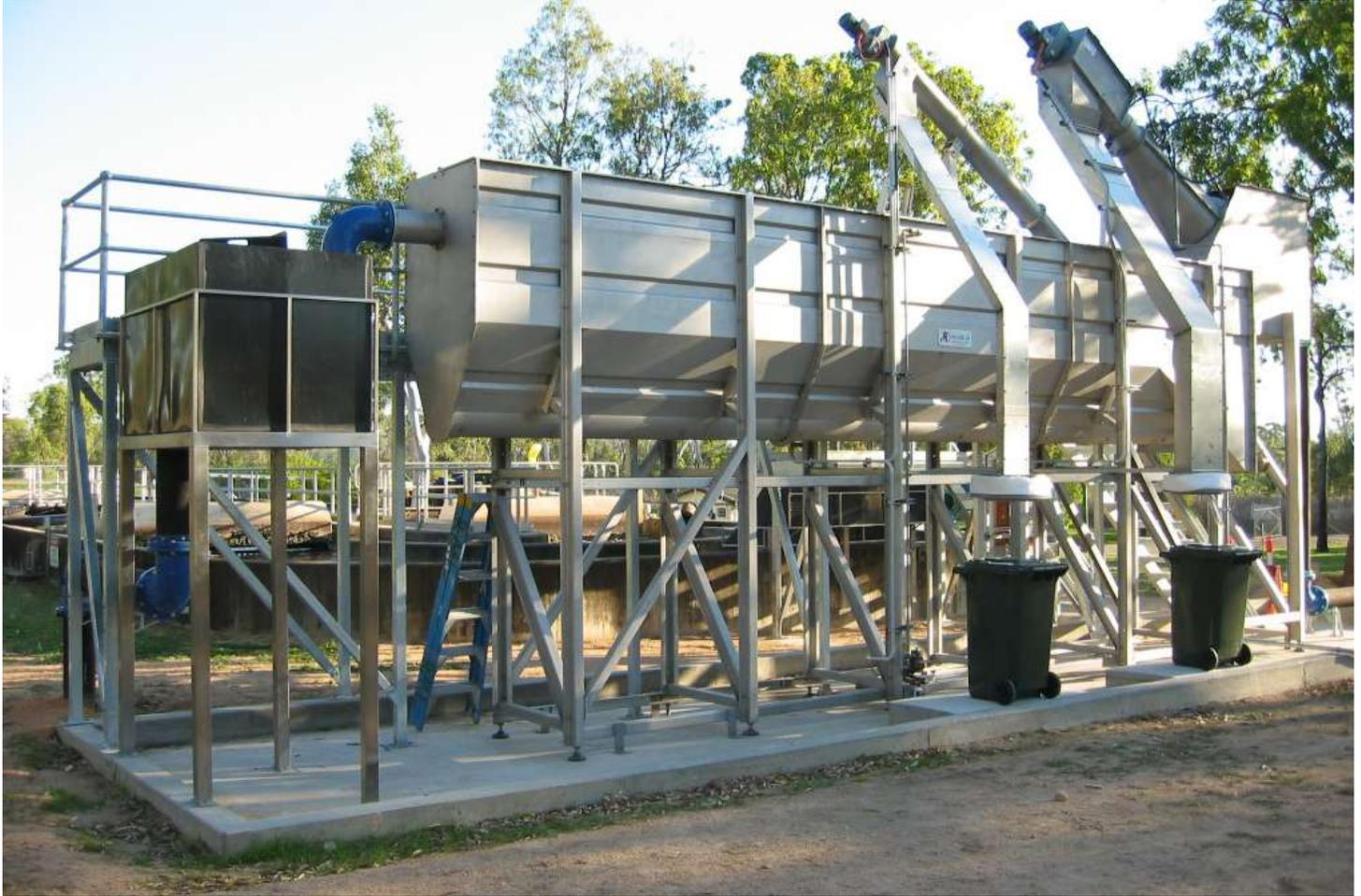
The Noggerath® Complete Headworks Unit (TOP) replace conventional headworks structures in wastewater treatment plants.
