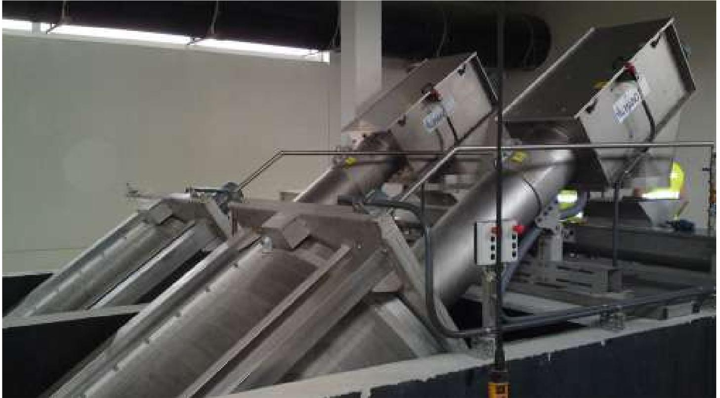
The Noggerath® Rotary Drum Screen (RSI) is a machine with a revolutionary drive concept. Contrary to conventional technology drives, the drum screen, via its discharge conveyor, drives the drum directly.
